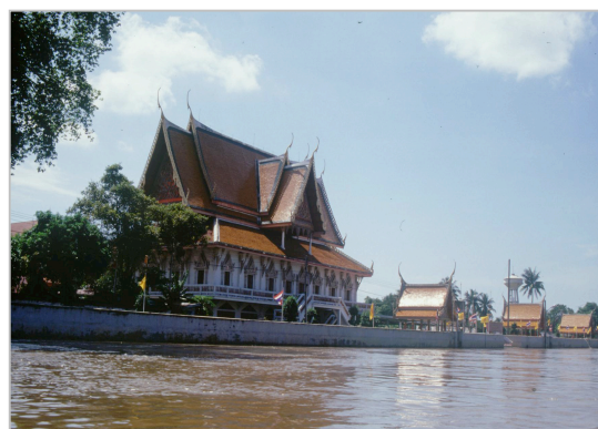
Fig. 16 The embankment deteriorates the magnificent view both from and to the river
